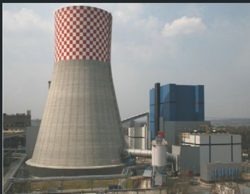
Figure 4: Łagisza 460 MW SC CFB power plant, Będzin, Poland
