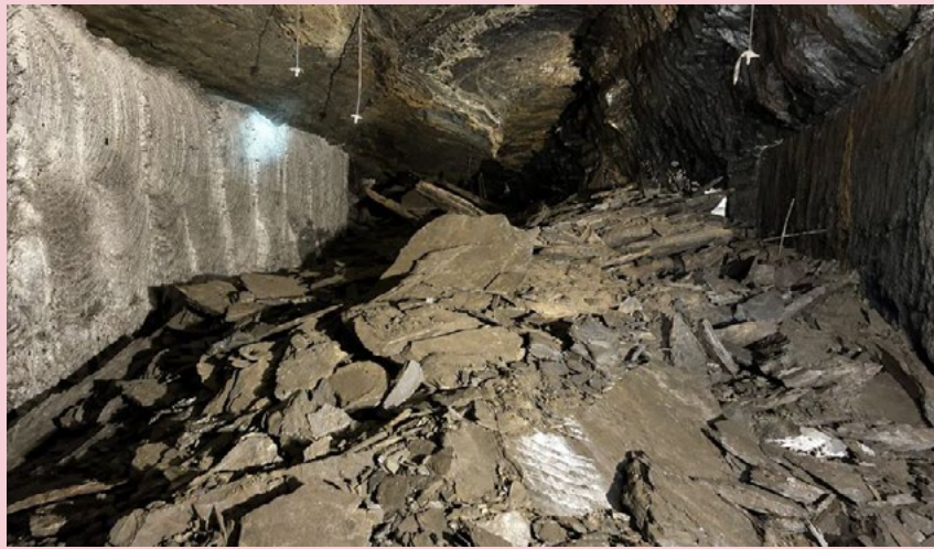
Potential impact of high horizontal stress in Coal Mines (Seriti Power)
