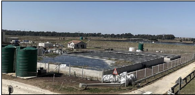
cloSURE ® demonstration plant, EWRP
