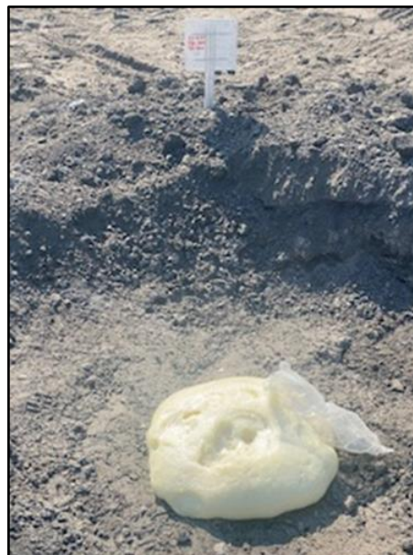
Figure 11: Foam expander plug on a hole collar
