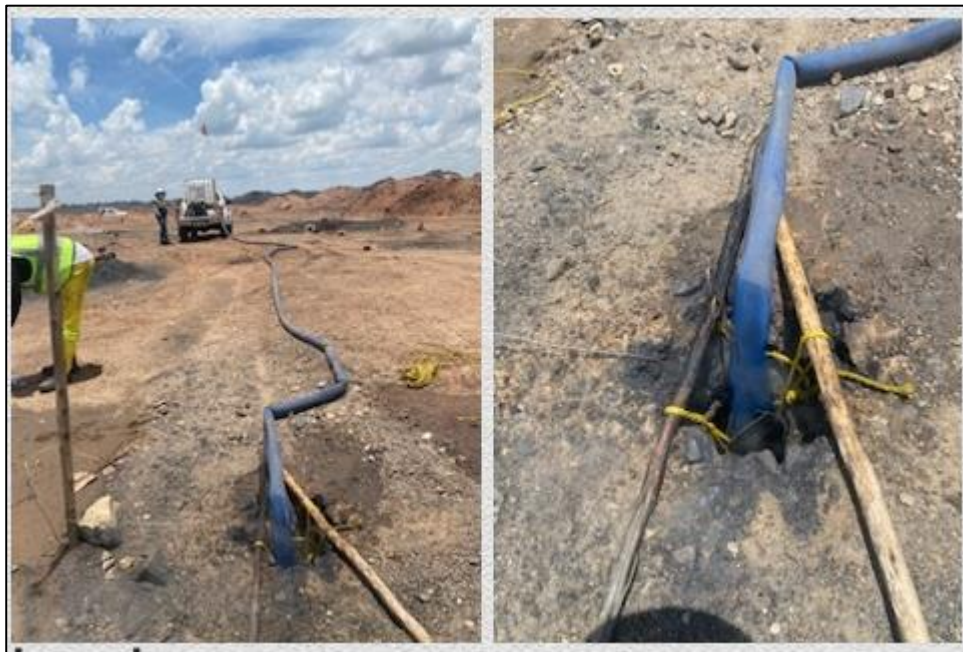
Figure 66. Pumping of water into the PVC sleeve in the hole
