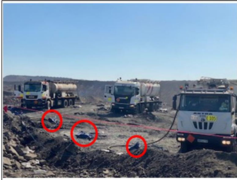
Figure 37: Sleeves placed next to hot holes before charging (circled in red)
