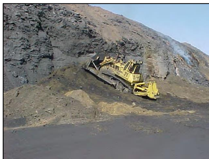
Figure 2. Dozing of a highwall with soil (Eroglu, 2003)
