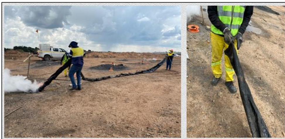
Figure 67: Retrieval of a PVC sleeve from the hole after the test
