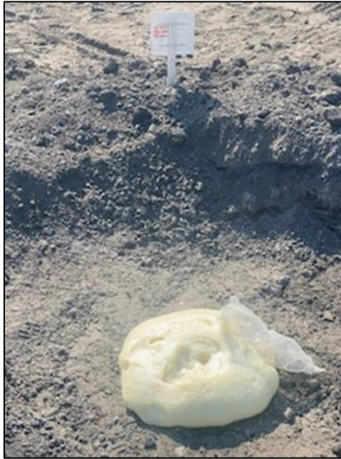
Figure 38: Foam expander plug used to close off a hot hole
