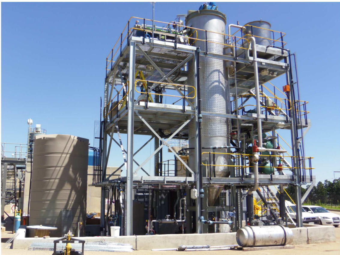
Figure 3.5: Optimum Colliery Prentec EFC pilot plant
