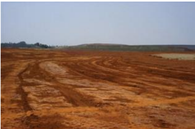
Highly compacted soil surface smoothed by a grader
