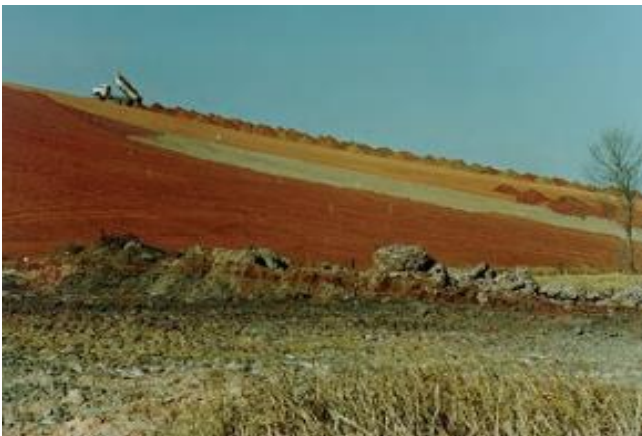
Replacement of topsoil
