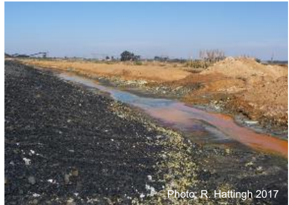
Coal discard dump toe seepage
