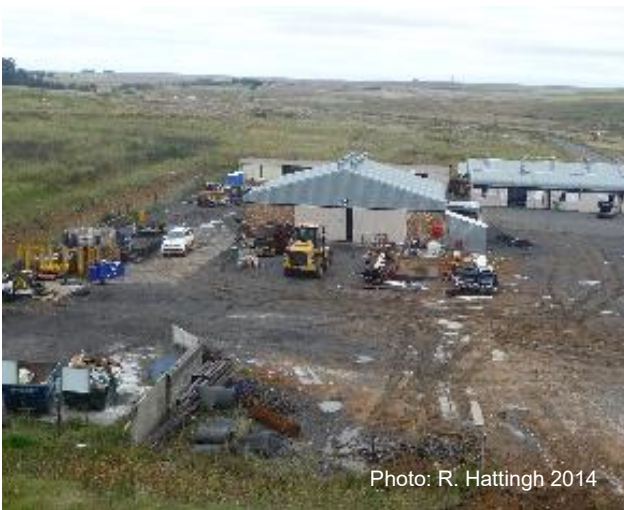
Contaminated footprint areas that require clean-up and remediation prior to shaping and revegetation as part of the site-wide landform design
