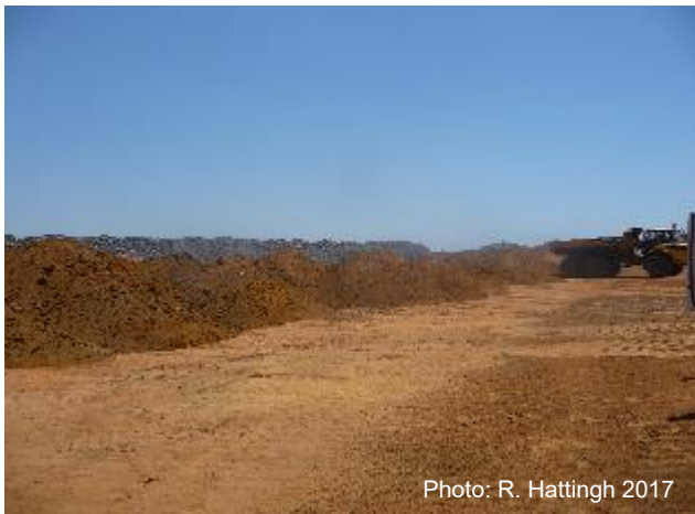
Topsoil replacement on back-filled spoils
