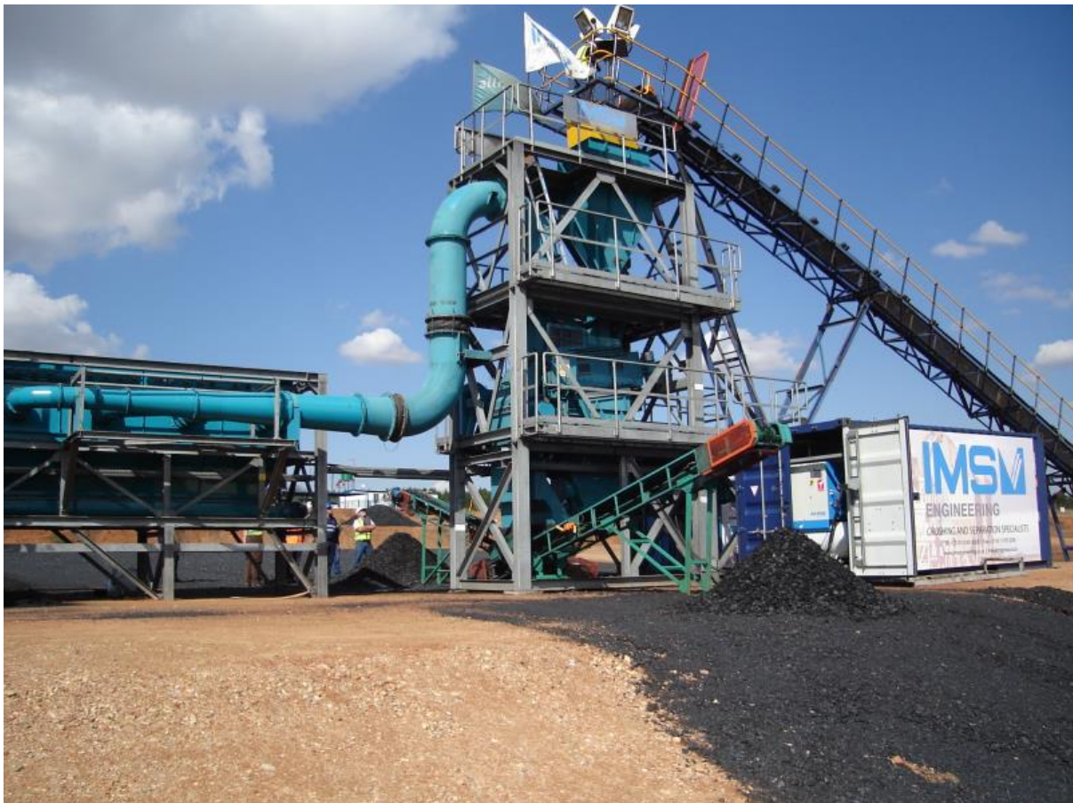
Figure 1: Allair jig at Slater Coal Marketing's Balmoral site
