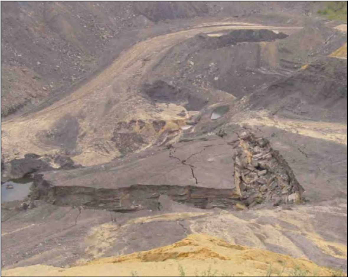
Figure 3.1.6: Wedge failure in hard overburden (photograph courtesy of New Vaal Colliery)
