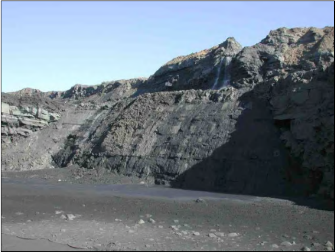
Figure 3.2.3: A failed highwall where the mode of failure was planar (photograph courtesy of Wonderwater Strip Mine)
