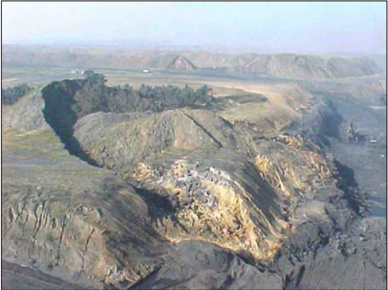
Figure 1.2: Highwall failure at New Vaal Colliery (photograph courtesy of New Vaal Colliery)
