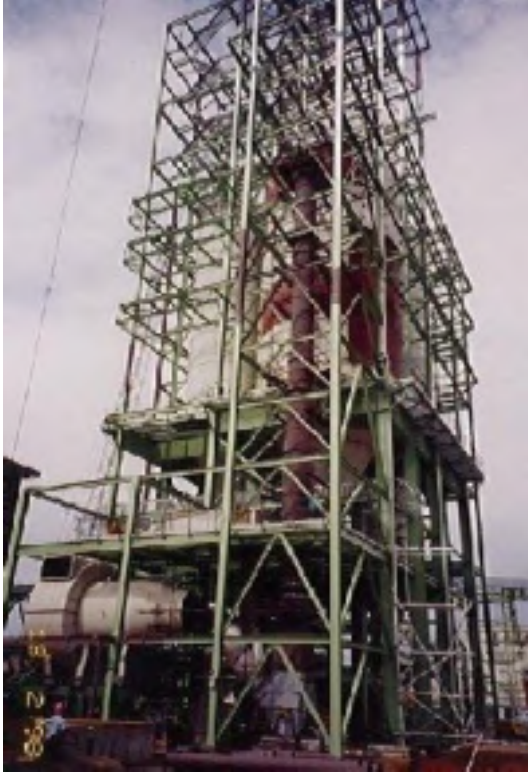
Figure 9: Flash dryer for chrome ore
