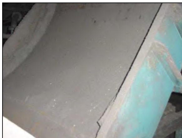
Figure 14: Sieve bend in operation
