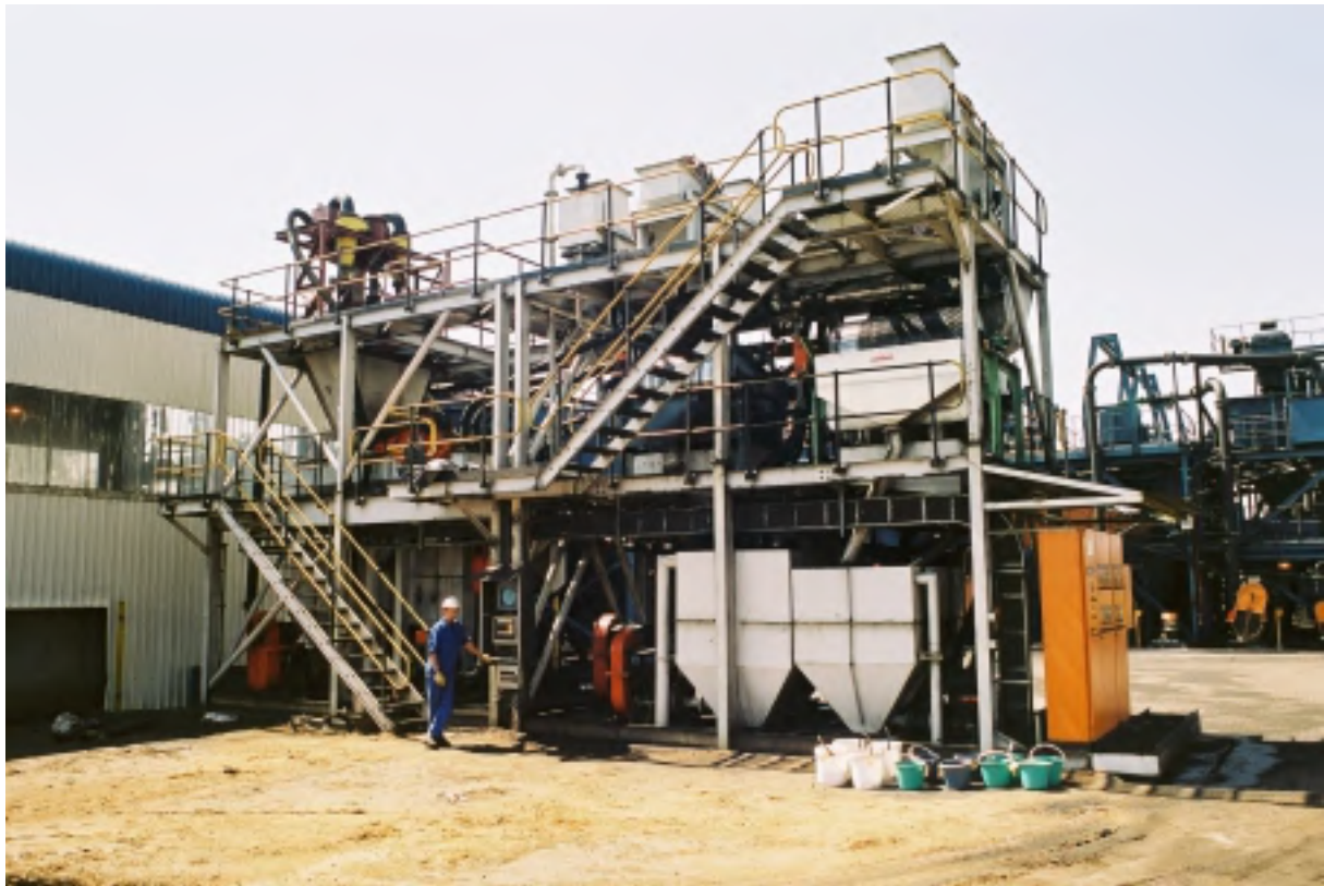
Figure 1: Photograph of the test plant at SWC
