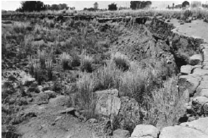
Figure 8-1 Collapse of a pillared area in the Witbank Coalfield
