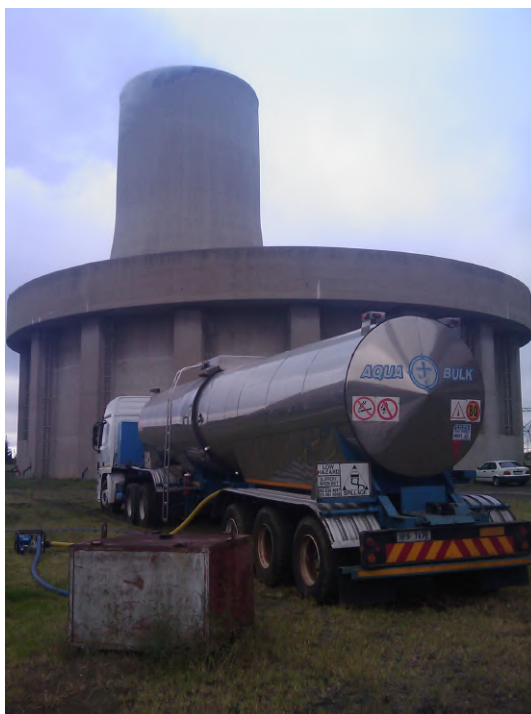
Figure 3. Collection of RO brine sample from Tutuka Power Station
