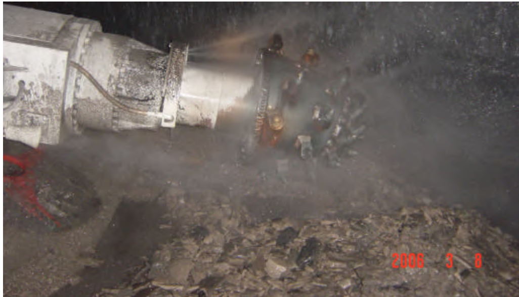
Figure 6: Cutting a sump into the sandstone floor
