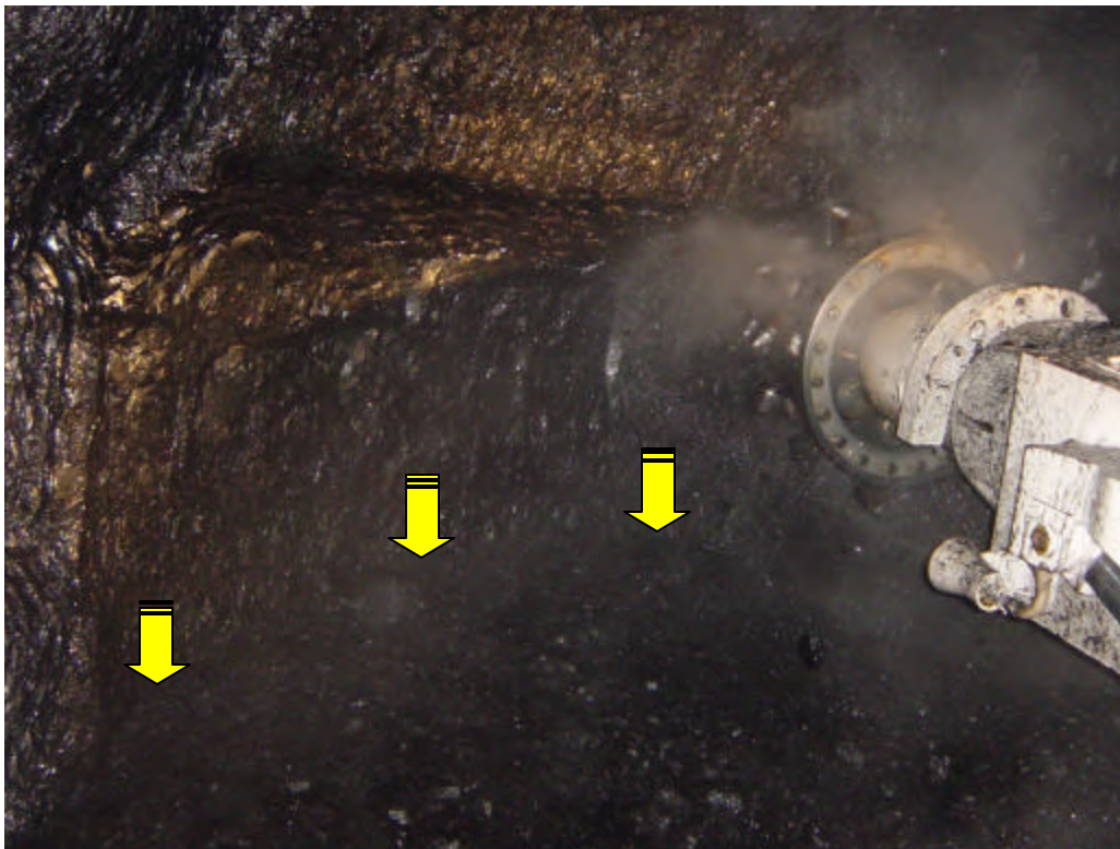
Figure 5: Muck pile forming below cutting head(below arrows)
